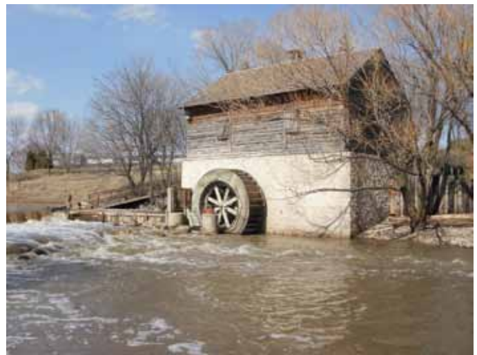
Grant’s Old Mill at 2777 Portage Avenue.
