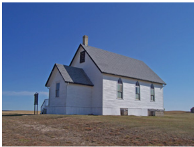
Construction Date: 1919 (RM of Whitewater) http://www.mhs.mb.ca/docs/sites/berbankchurch.shtml
