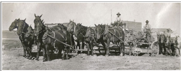
Locals found work grading the line.
