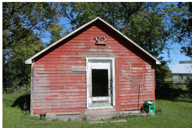
This building, once a fertilizer shop in Rivers, was purchased from Bob McLaren. It served as the first "General Store" and was later known as "The Jug House"
