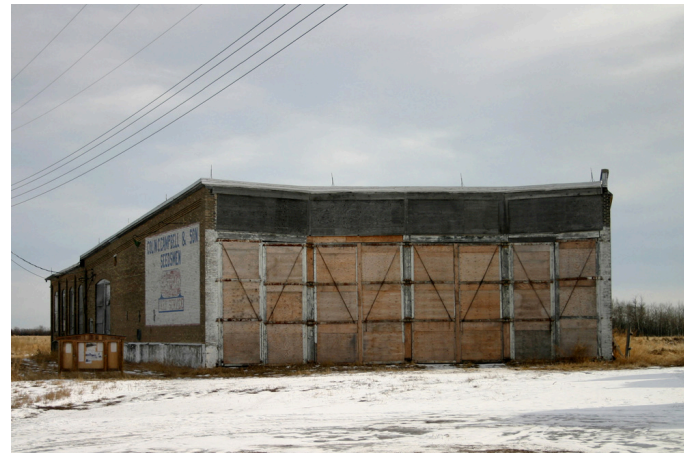
Reston CPR Engine house in 2008
