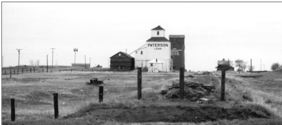
Lena – after the railway was abandoned.
