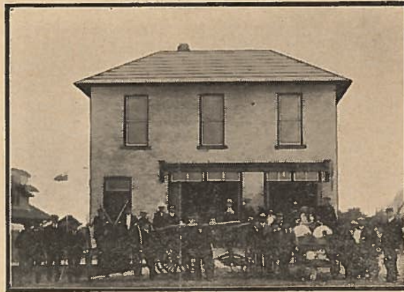
DELORAINÉ FIRE HALL AND BRIGADE.
