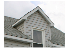
Gable roofed wall dormer – window flush to wall, not set into the angle of the roof.
