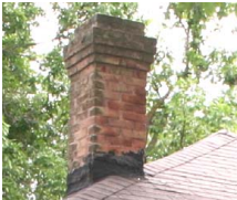
An original brick chimney with its attractive silhouette.
