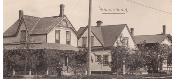
Most homes had two chimneys, but few remain in Hartney today.
