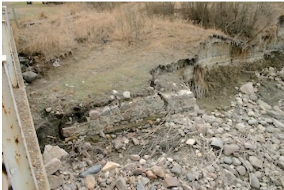
High water in 2012 exposed the abutments of the previous bridge.
