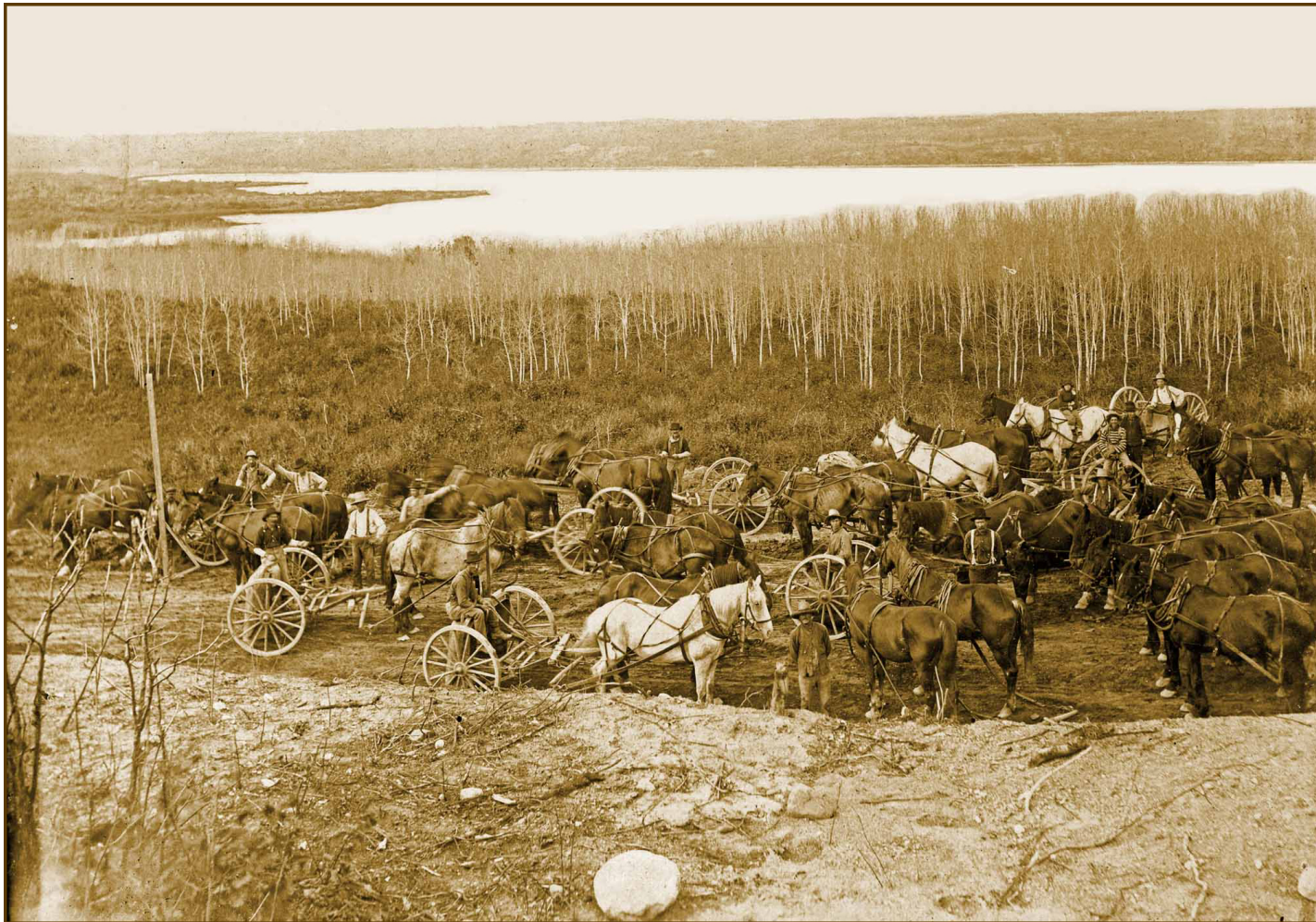
Grading the "Wakopa Branch" near the site of Neelin, with Lake Louise in the background.
