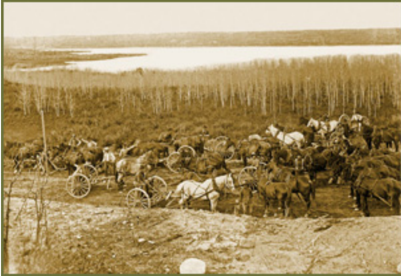
Grading the line near Neelin (James Wall Collection - McKee Archives)
