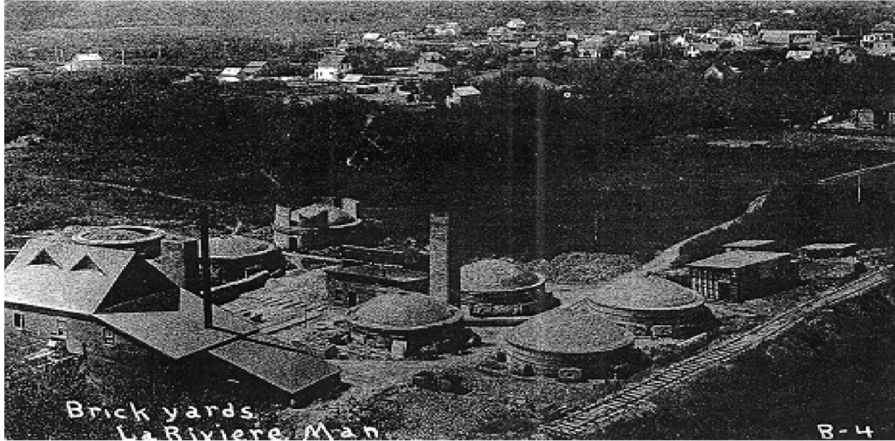
LaRivière Brick Plant, c1903. The large kilns are very prominent in this view, along the crusher building at the left. (LaRivière historical Book Society. Turning Leaves, A History of LaRivière and District . Altona: Friesen, 1979. Front endpapers.)
