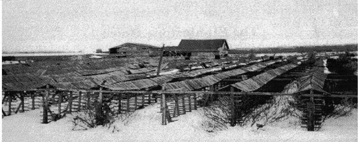
Brick drying racks, Virden Brick Yard. ( Anecdotes and Upgrade, 1882-1982, Virden Centennial Souvenir. Virden: Empire Publishing Company, 1982. p. 29.)
