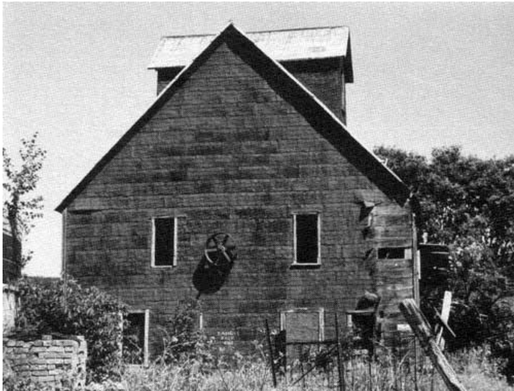
Brick plant at Leary's, 1989 (David Neufeld)
