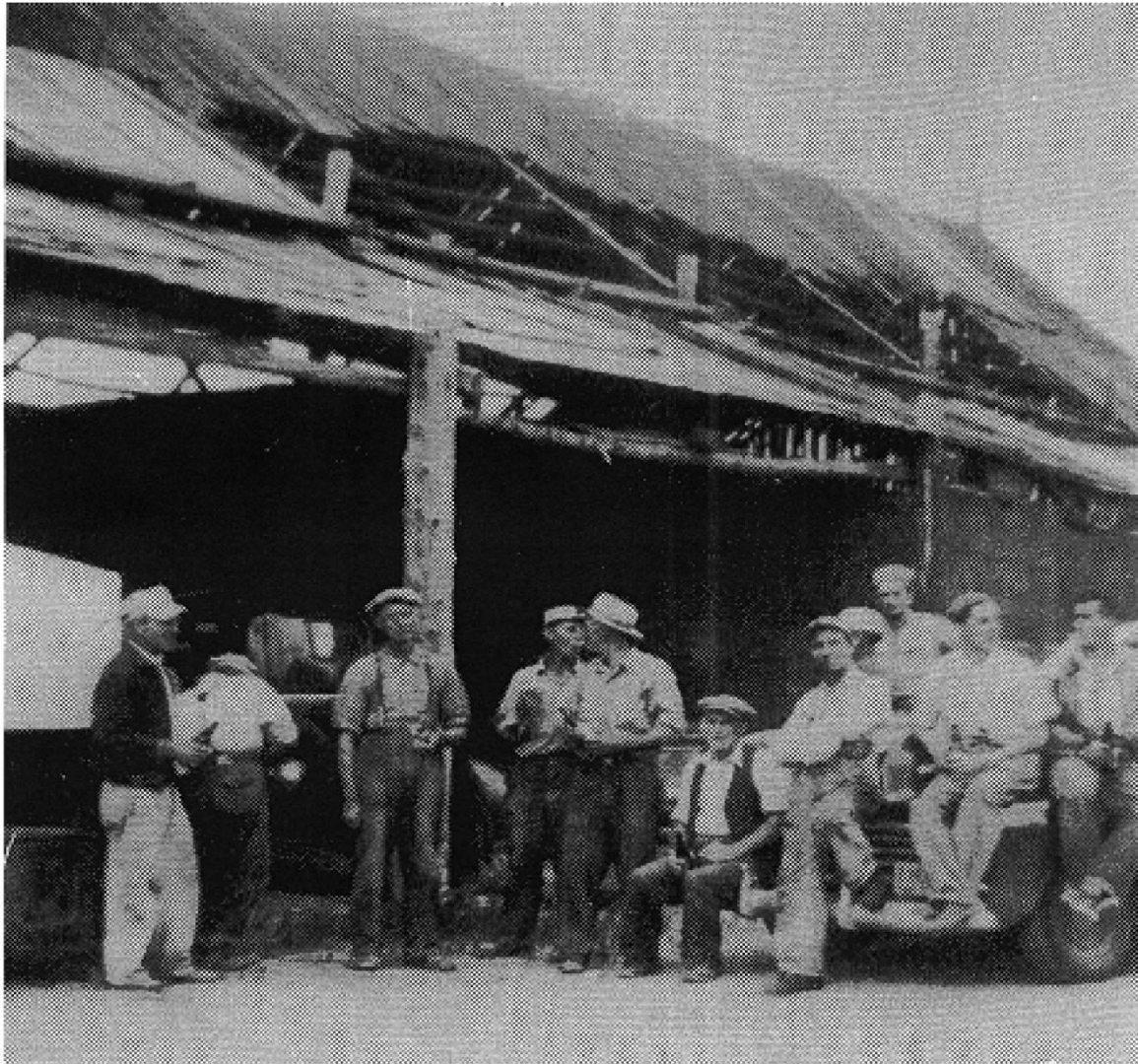
Kiln shed with kiln in rear, along with open roof, Whitemouth Brick Yard. (Bob Porth and Craig Mackenzie, eds. Tails to Rails to Highways . N.P.: Whitemouth Municipal Museum Society, 1979. P. 102.)
