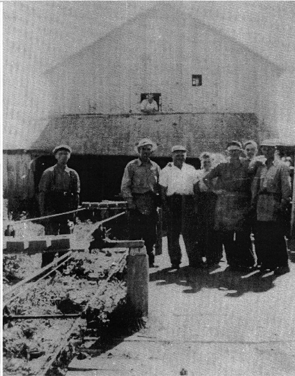
Main Building and portion of brick conveyer, Whitemouth Brick Yard. (Bob Porth and Craig Mackenzie, eds. Trails to Rails to Highways . N.P.: Whitemouth Municipal Museum Society, 1979. P. 101.)
