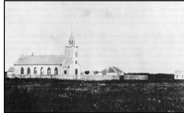
Figure 19. First church of St. Paul's, Middlechurch, 1876. (PAM)
