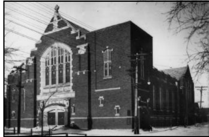
Figure 54. St. Matthew's, Winnipeg, 1912. (PAM)
