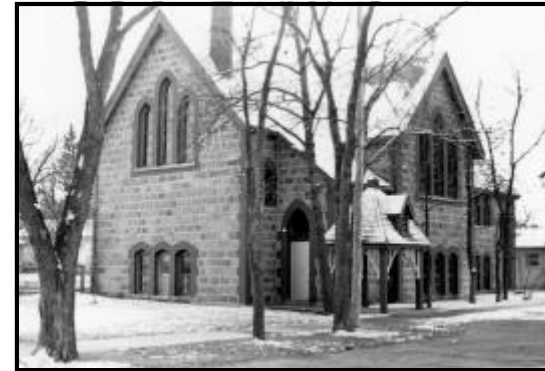
Figure 59. St. Mark's, Minnedosa, 1903-04.
