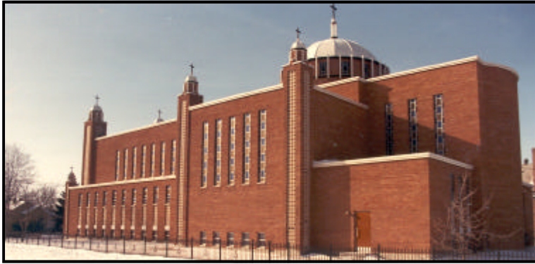
Plate 67. Blessed Virgin Mary Church. The cruciform plan is evident here and the dome is an important element of the design. The chancel is integrated into the main body of the building. Although the elements are reinterpreted, the large massing characteristic of Ruh's churches is present in Deneka's design.
