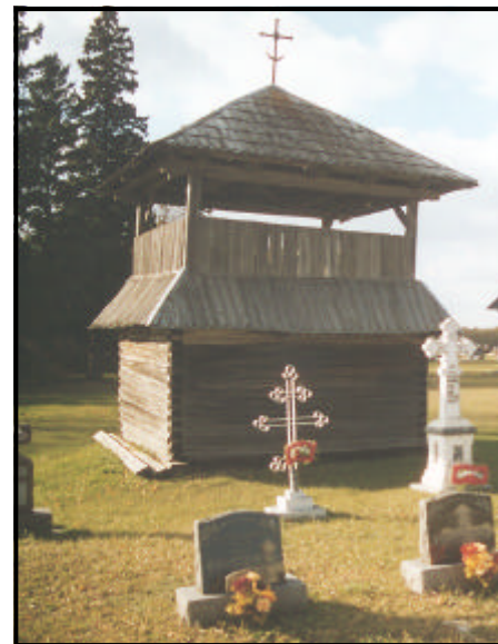
Plate 26. Bell tower of St. Alias church, Sirko. The roof of the tower is built of roughly laid vertical shakes similar in nature to planking. Bell towers were a ubiquitous feature on Ukrainian churchyard in Manitoba, just as they had been in Ukraine. Those in Manitoba were, like this one, simply constructed and animated with a few functional, but decorative elements.
