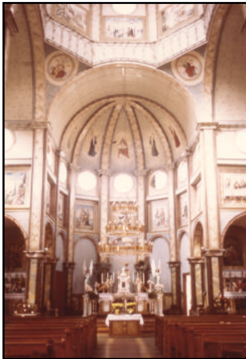
Plate 56. Church of the Assumption, Portage la Prairie. View of the central crossing. Also visible is the apsidal form of the chancel with its half dome and the barrel vaulting of the nave and transepts.
