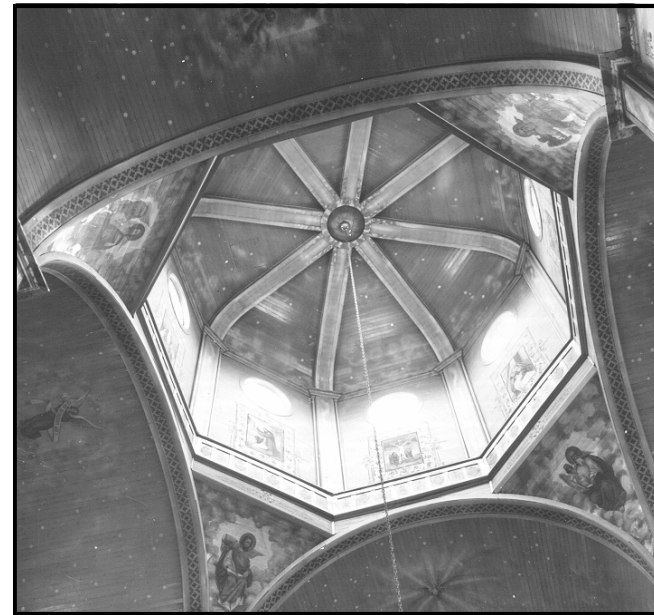
Plate 53. St. Mary's Church, Mountain Road. Each of the pendentives beneath the dome had a figure painted on it. (Provincial Archives Manitoba)
