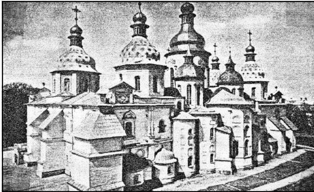
Plate 11. St. Sophia, Kiev. The central five apses of the original eleventh century structure form the nucleus of the enormous seventeenth century structure. The present exterior is almost entirely the result of additions in the Ukrainian Baroque style (D. Buxton, Russian Medieval Architecture, Plate 57)
