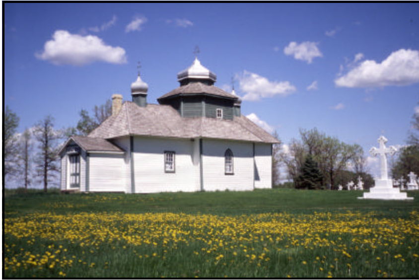
Plate 19. St. Michael's Ukrainian Greek Orthodox Church, Gardenton. The Plan of the church – three frames oriented on an east-west axis with the central frame slightly larger than the adjacent two – has remained basically unaltered.
