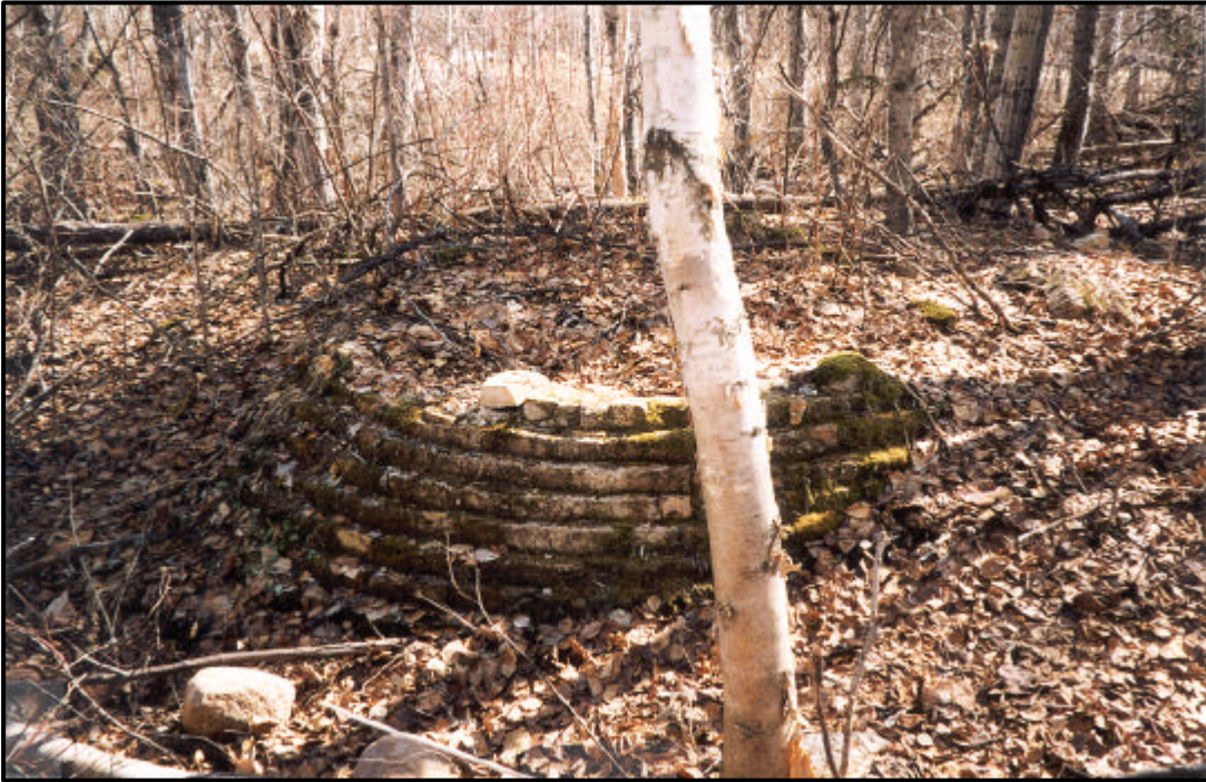
Remnants of refuse stack used to burn the bark and trimmings at the Red Deer Lake mill, 1998. The fire transformed water into steam to power the sawmill. Source: HRB.
