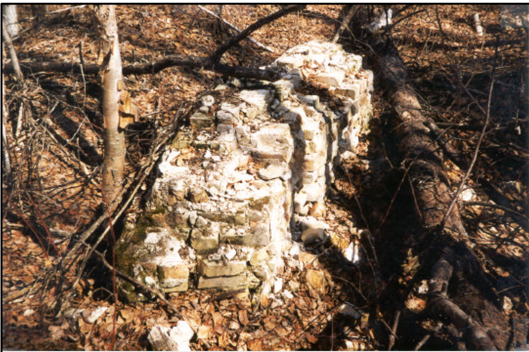
Remnants of cement footings along Red Deer Lake, 1998. Probably supported the jack ladder that carried the logs from the lake shore to the sawmill. Source: HRB.
