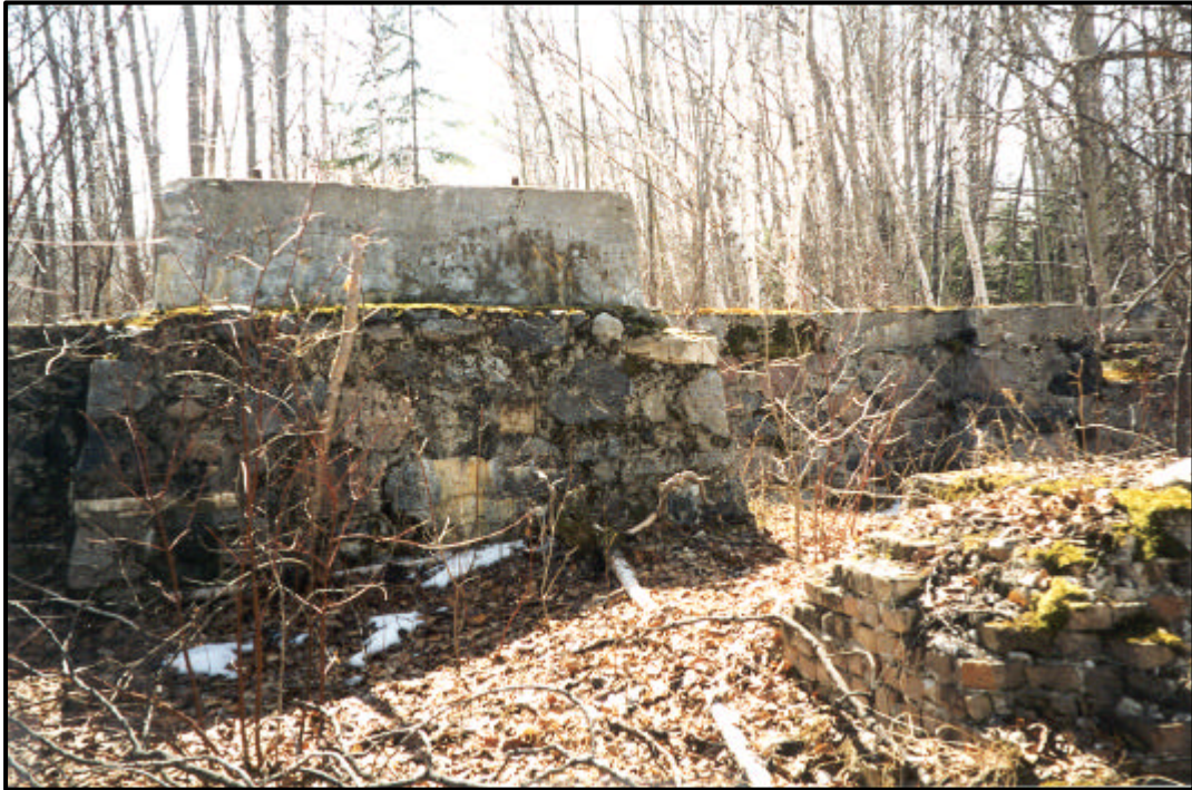
Remnants of the foundations that supported the steam engine used at the Red Deer Lumber Company mill at Red Deer Lake, 1998. Source: HRB.
