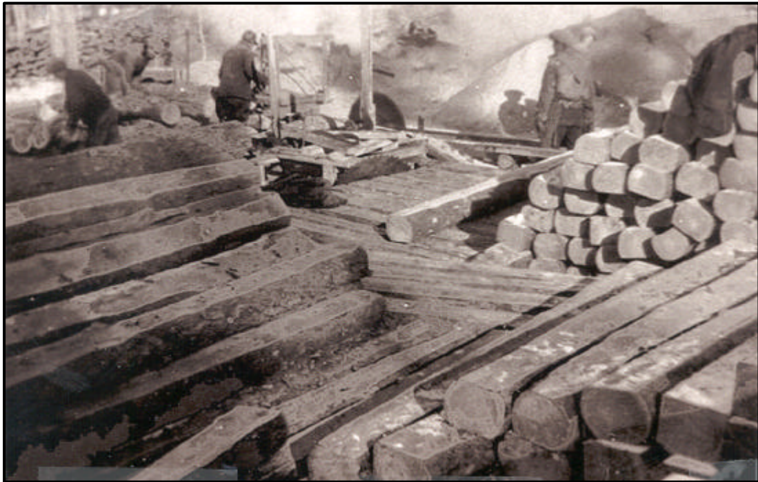
Cutting railway ties at a sawmill at Montago Lake, northwest of Fisher Branch, 1941. Source: M.Roche.
