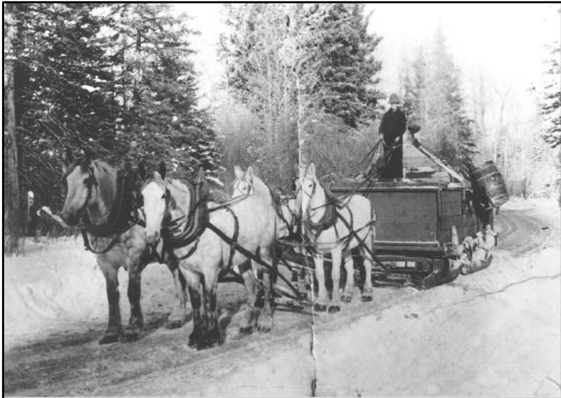
Water sleigh used to create the ice roads used in lumber camps, c. 1906. Source: P.A.M.
