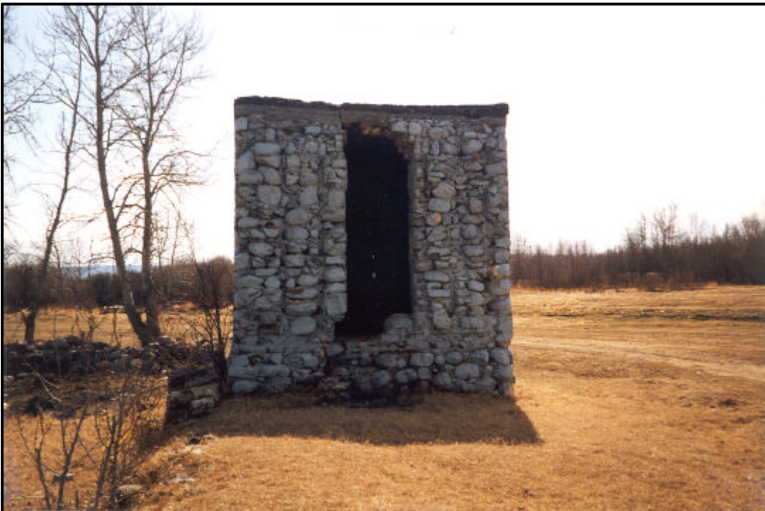
The remains of the vault that once stood in the offices of the Red Deer Lumber Company, 1998. Source: HRB.
