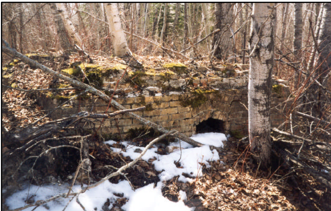
Remnants of the stack used for heating the water to power the steam engine at the Red Deer Lake mill, 1998. Source: HRB.
