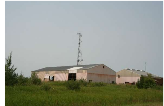
View in 2017 of the brick-pressing building and main offices of the Red River Brick and Tile site near Lockport.
