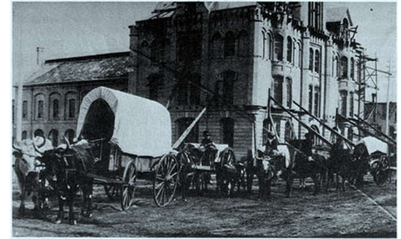
Shoring-up Winnipeg’s City Hall, which would come down in 1883, just seven years after it went up, in 1876. (Courtesy Archives of Manitoba)
