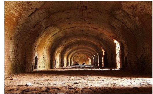
Interior view of a continuous kiln, with partition walls removed. (Courtesy Wiki-Commons)
