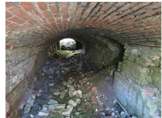
A brick-lined drying tunnel, one of the few remnants of the Sidney Brick and Tile operation, seen in 2013. (Courtesy Manitoba Historical Society)
