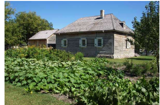
The Ross House (1852), now a museum in Winnipeg, at one time served as the post office for the Red River Settlement. It was typical of house construction of the era – seen here with its log walls, wooden shingles and the one brick feature: the chimney.
