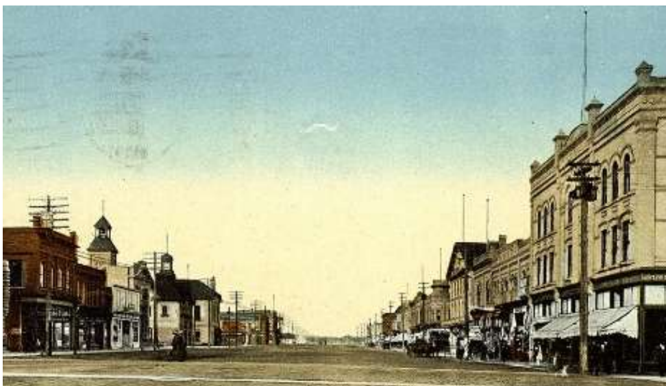
A postcard view of Portage la Prairie's main commercial thoroughfare, Saskatchewan Avenue. (Courtesy University of Alberta) The view suggests the wealth of brick buildings rising in nearly all Manitoba communities. Doubtless it would have been from W.P Smith's local yard that much of the brick seen here would have been pressed and burned.
