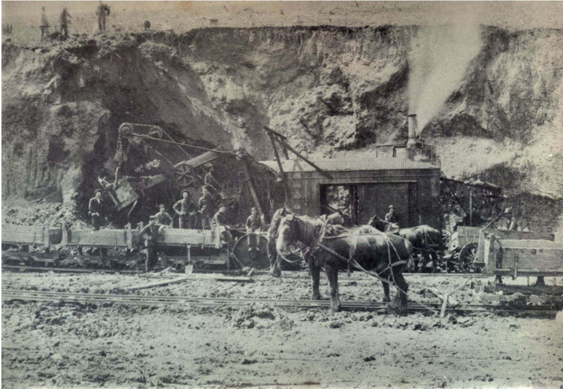
THE STEAM SHOVEL EXCAVATES AND THE HORSE-DRAWN DUMP-CARS HAUL AWAY the fill on the bench on the south side of the Souris River valley about 1905. Photo Gilford Copeland
