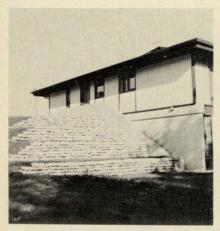
If large differences in grades have to be retained, it is advisable to create a series of smaller walls, each set back to create terraces. instead of one high wall.
