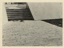
Another application of Tyndall stone is the use of material pre-cut in 6" - 8" strips of different length.
