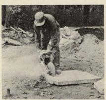
If narrow joints are desired, Tyndall stone may be cut on the construction site and fitted closely together
