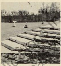
Each stone layer of the retaining wall is terminating level with a step of this Tyndall stone stairway.
