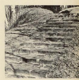
A rustic but safe stairway, blending well into the landscape. Split granite, laid in concrete, has been used with steps protruding above the face of the slope.
