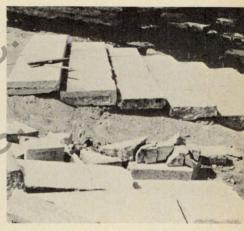
A Tyndall stone stairway under construction. Shallow risers and long treads as shown are highly desirable for outdoor steps.
