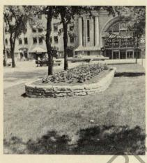
Most important for all wall or planter construction is the placing of perfectly horizontal layers. On this sloping area, three layers of stone are visible on the right side of the planter, while four layers can be seen on the left side.
