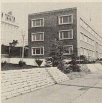
A well built, stable retaining wall of Stony Mountain limestone. An interesting effect is achieved by using a setback of 3" for each layer.
