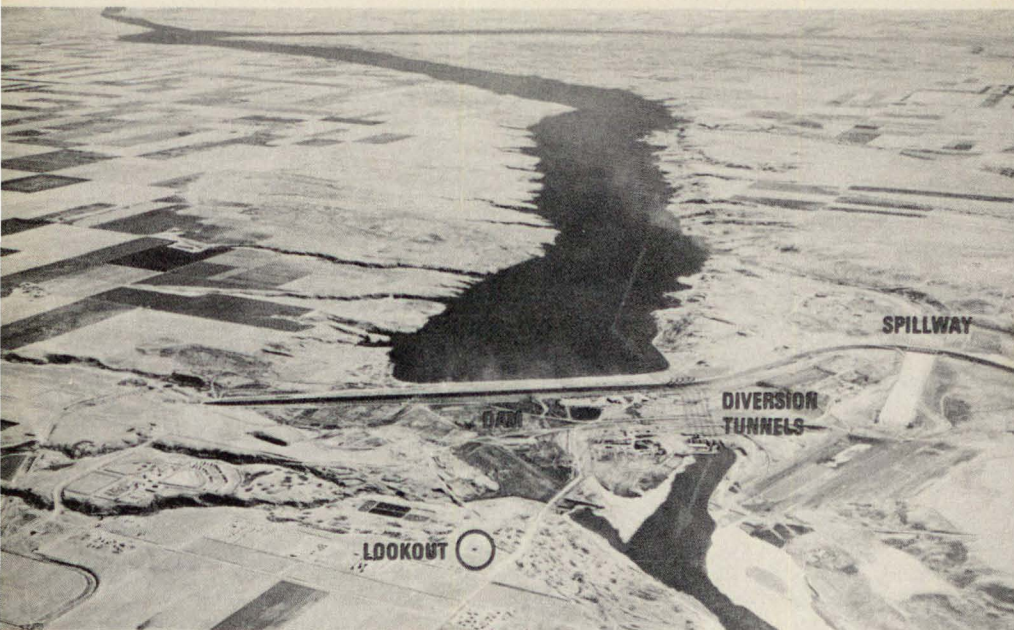
Profile of the Dam — showing earth construction, diversion tunnels and related structures.
