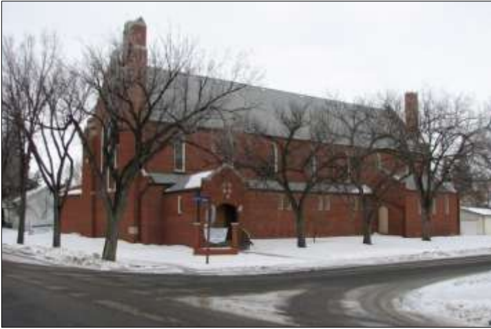
Church: view facing NE
