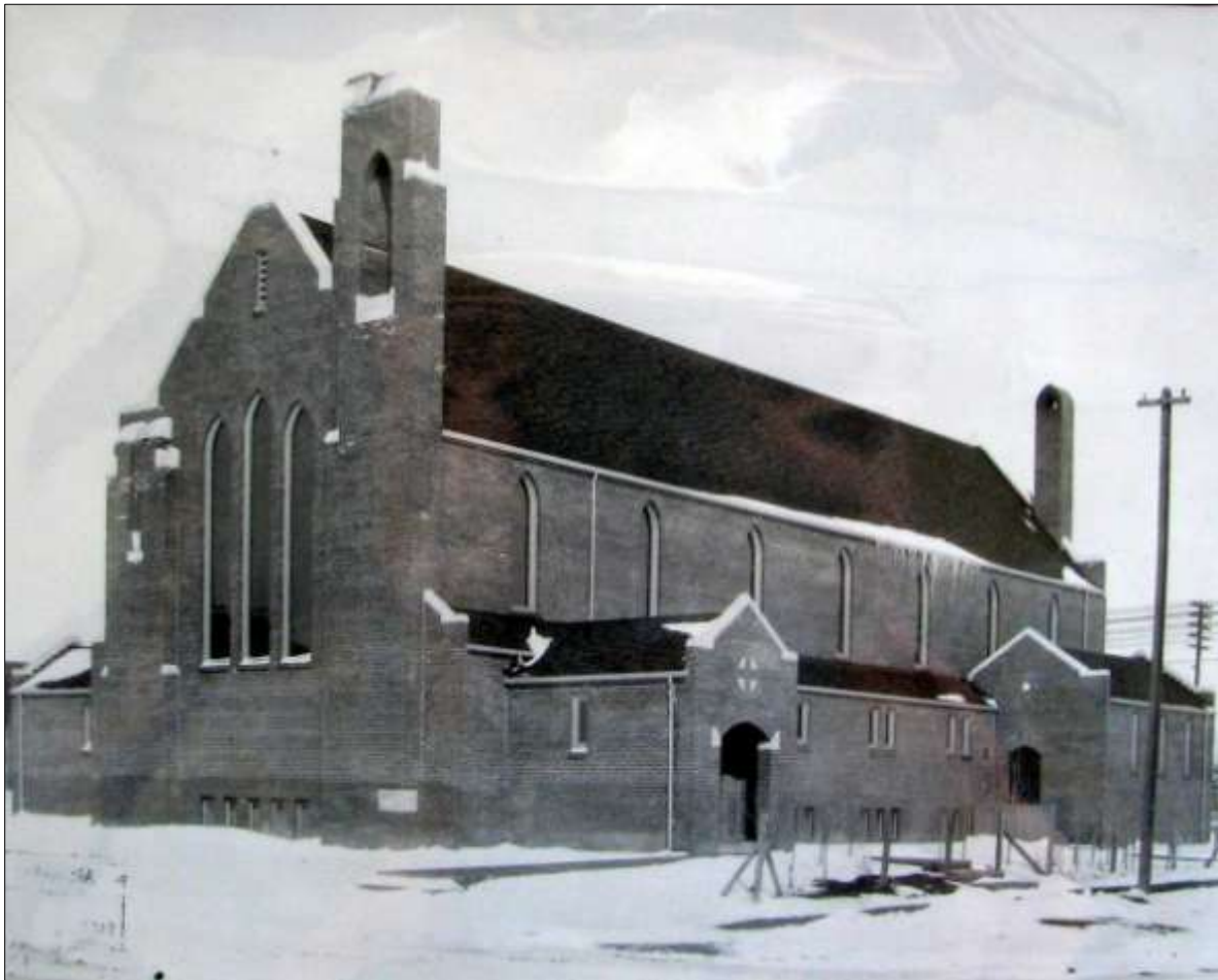
St. Mathew's Anglican Church shortly after completion in 1926.
