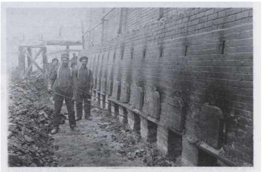
(Left) Tossers and setters stack bricks inside a scove kiln before firing c. 1910
