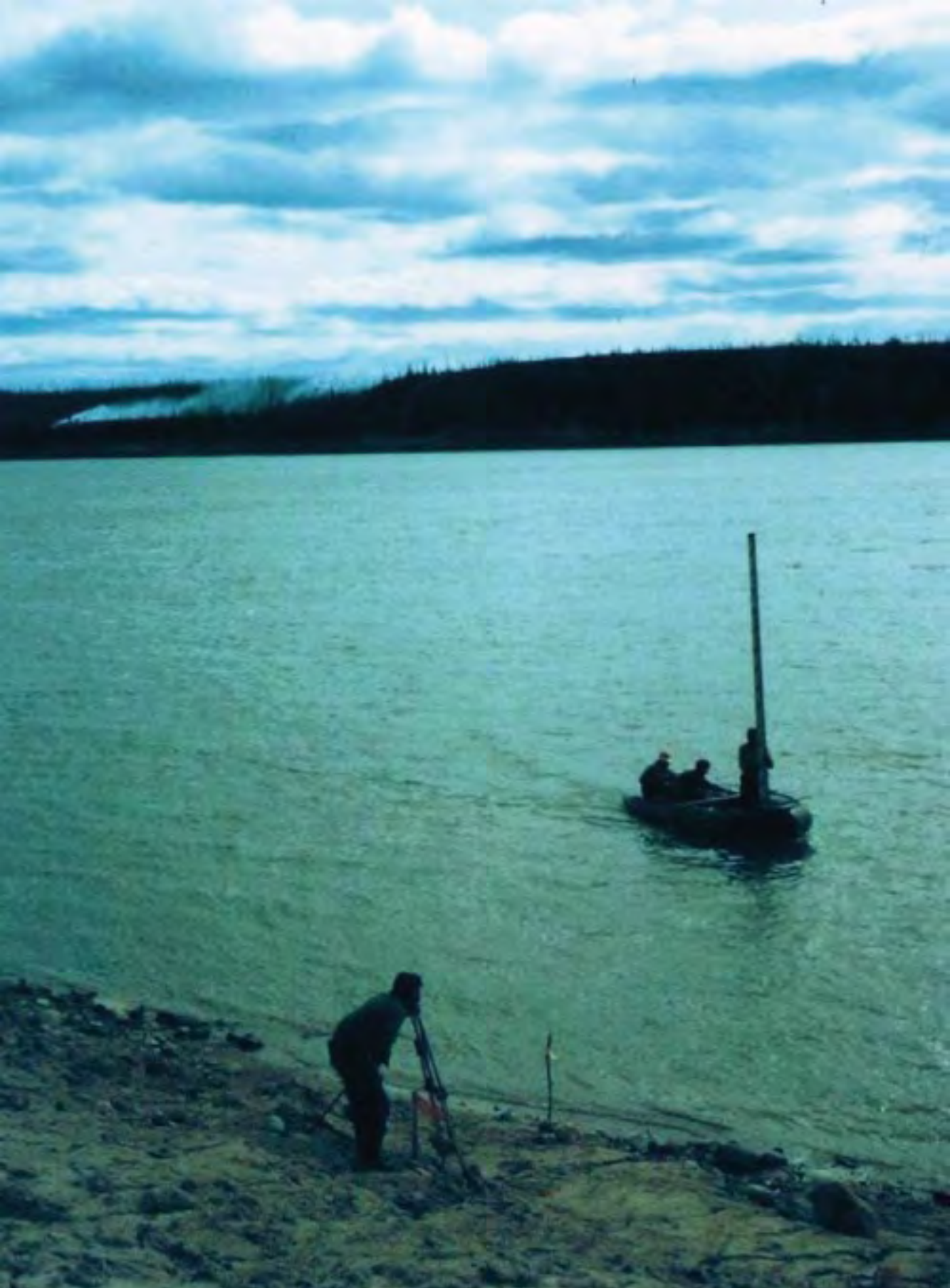
Depth-sounding crew at work — note stadia board in the boat and transit surveyor on shore
