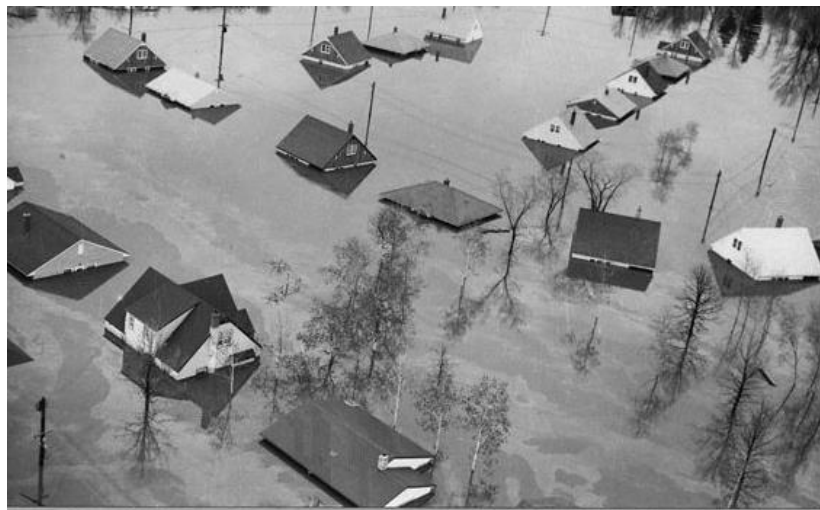
Tribune Photo by G. Aikman Figure 12. WILDWOOD PARK DISTRICT Wildwood Park district was one of Greater Winnipeg's most hard-hit suburbs. Many houses were submerged up to their roofs.
