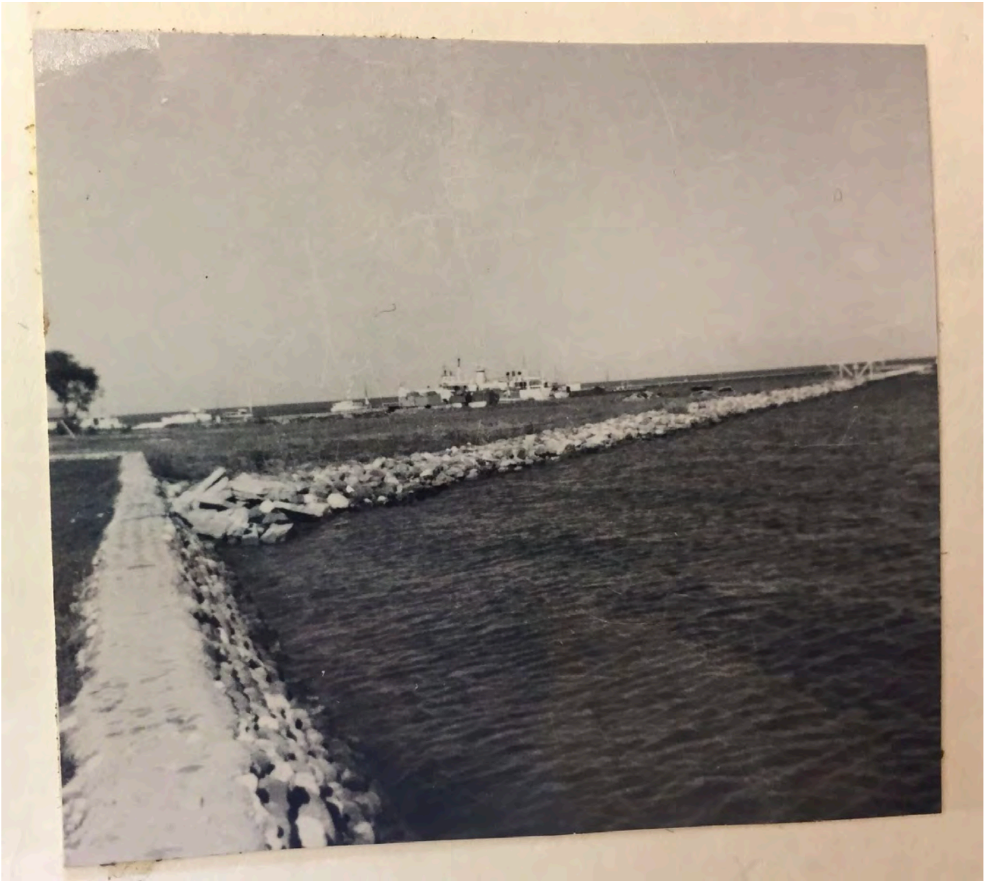
Protecting the harbour, looking northeast.
