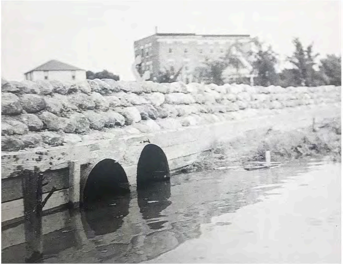
Looking north, finished breakwater in front of Betel Home, pre 1967.
