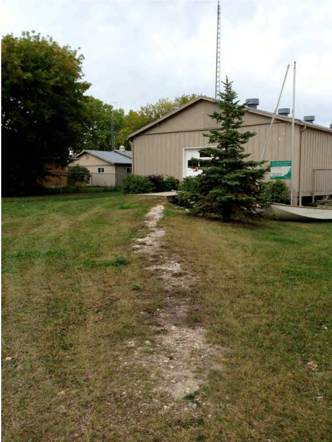
Ultimate north end of breakwater running into, and probably underneath, the Gimli Yacht Club locker (photo E Ward.)
