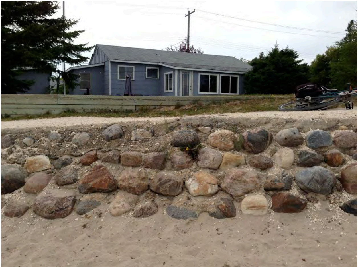
Breakwater wall, original section 2016 (photo E Ward.)
