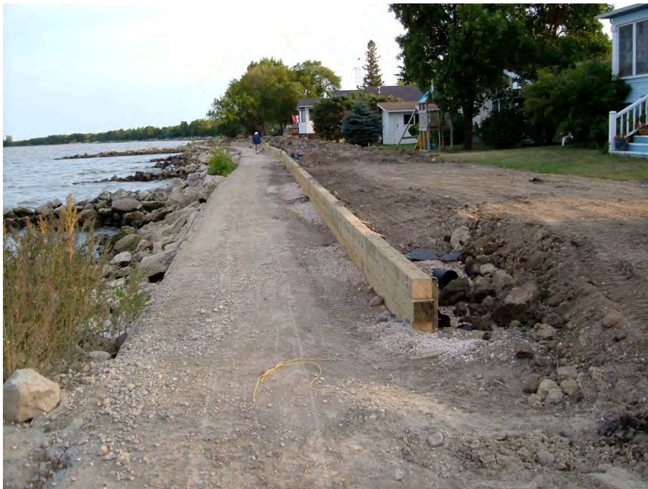
2006 construction (photo E Ward.)
