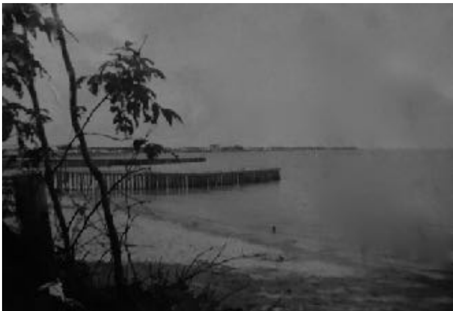
Wooden groins, ca. 1950s
