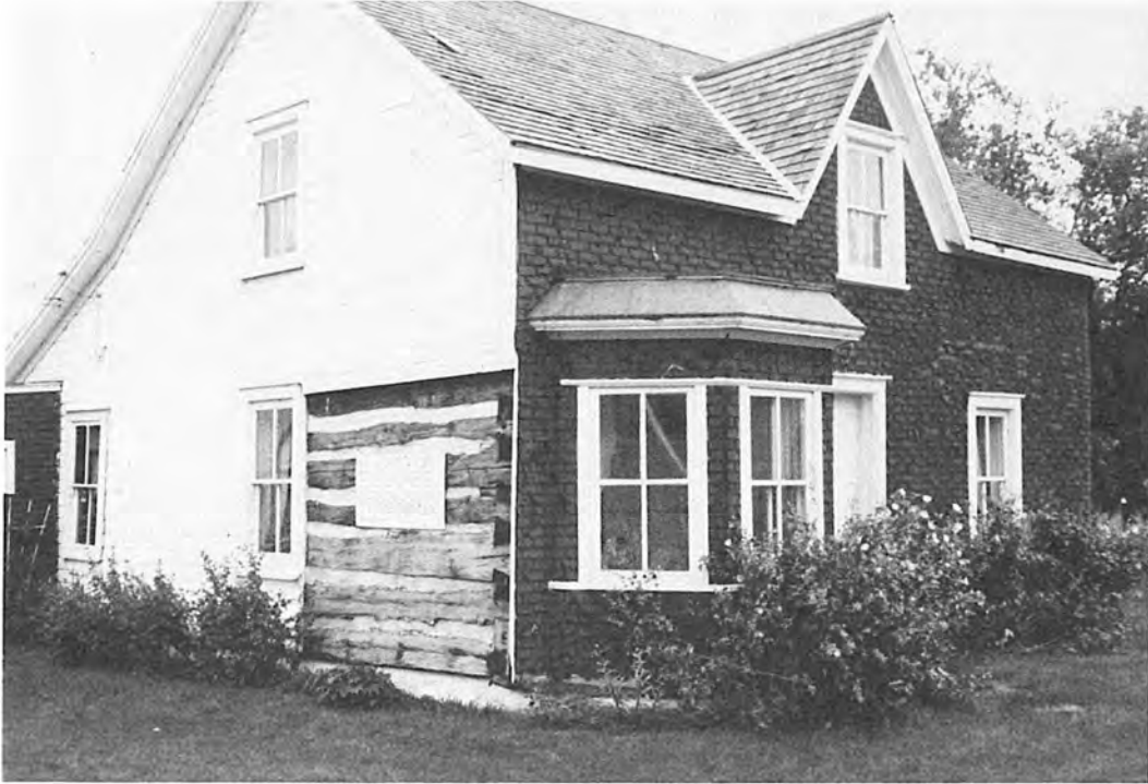
Log house, built in 1878 by William Hasselfield, where Nellie Mooney boarded in 1890-91 when she taught at Hazel school. A portion of the siding has been removed to show the dovetailing of the logs.
