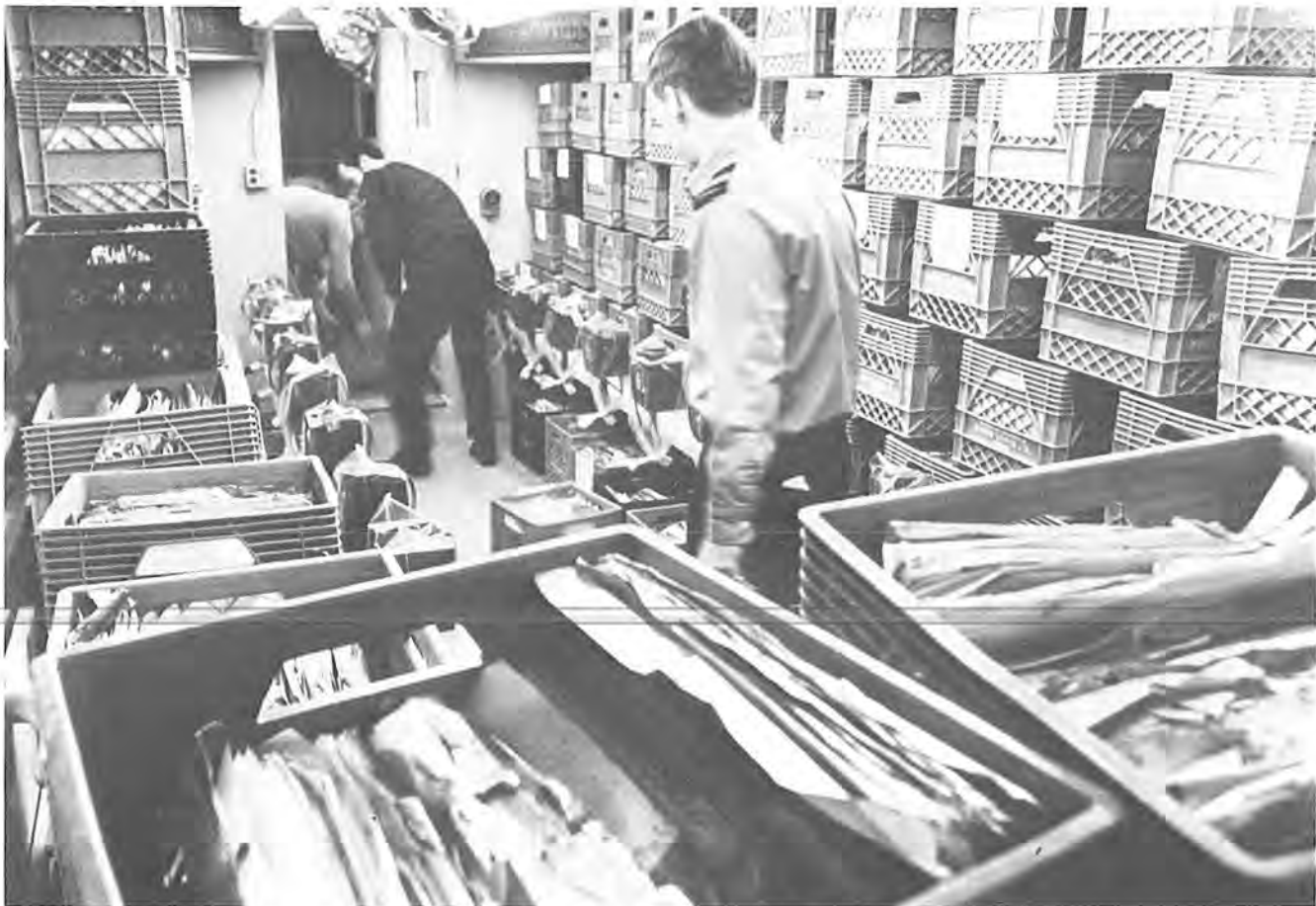
Crates of documents being placed in the chamber. Note the method of stacking the crates so as to allow maximum air circulation. Winnipeg Free Press
