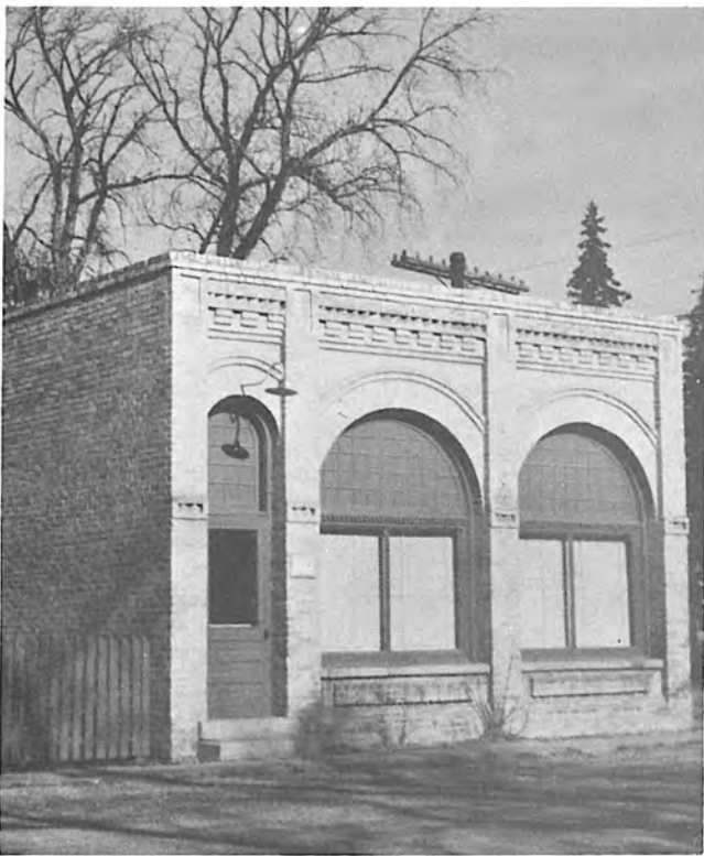
Oak Lake telephone office of brick
