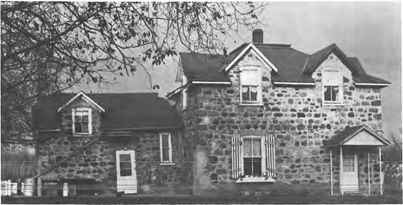
Fieldstone house, built by Lord Elphinstone in Virden, 1881, demolished 1974
