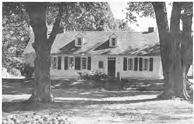
Perkins House in Liverpool, N.S. The home of merchant, ship-owner and diarist, Simeon Perkins, built in 1766.
