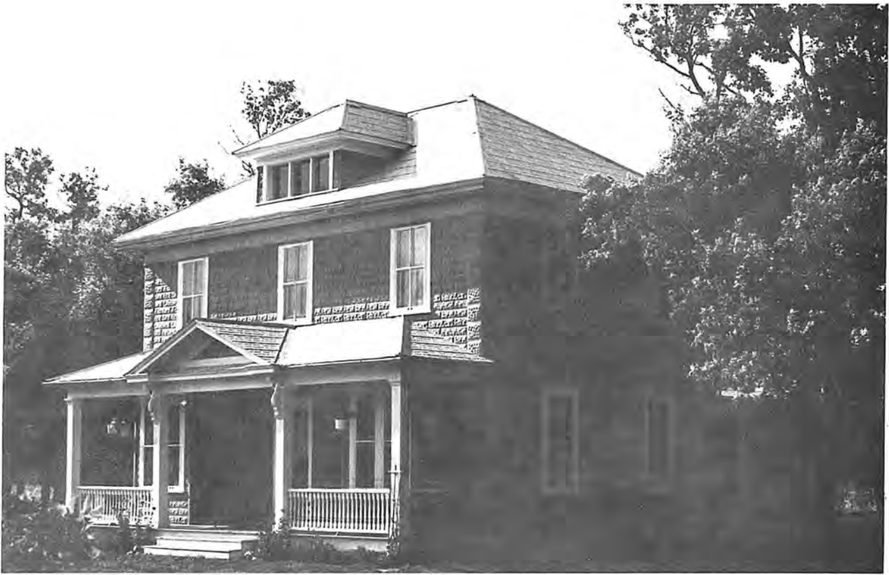
The "tin house" built by J.J. Wilson and now located on the grounds of the Archibald Historical Museum Y. Tessier
