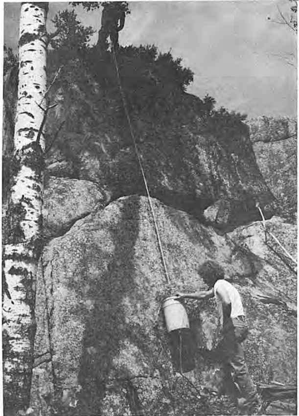
Hauling water for plaster
