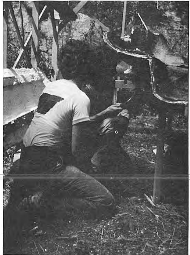
Nailing wood supports under the mold
