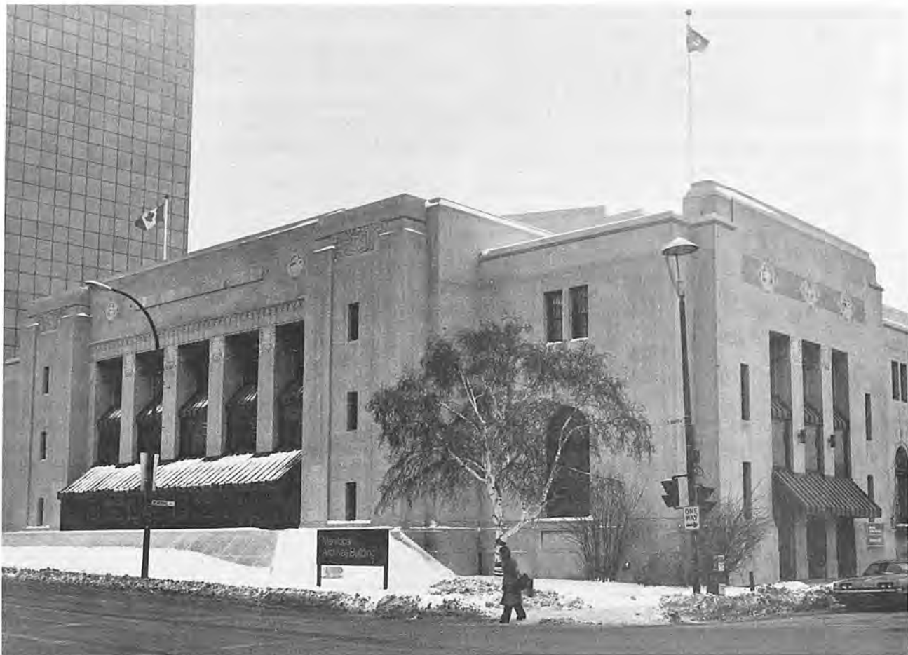
Exterior view of the Manitoba Archives Building
