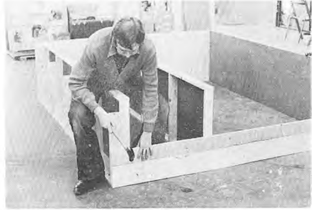
Figure 3 - Sides of rough lumber are nailed onto the shelves
