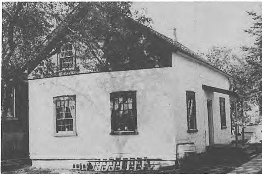
"Old Log House" before and after restoration
