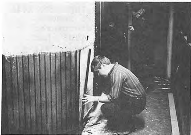
Removing wainscoting from the Bank of Montreal
