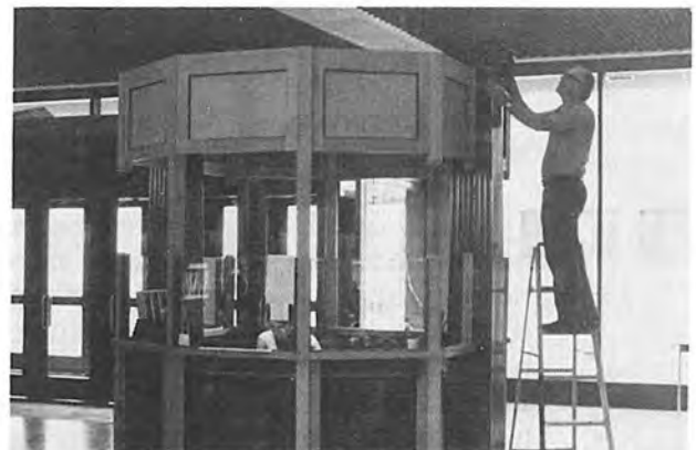
Telephone/Information Kiosk near completion
