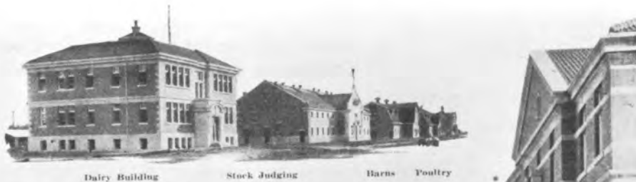
29. Manitoba Agricultural College - Fort Garry Site just after construction
