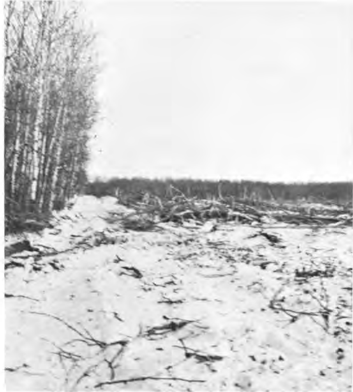
56. Brush knocked down by ball and chain in winter period 1963
