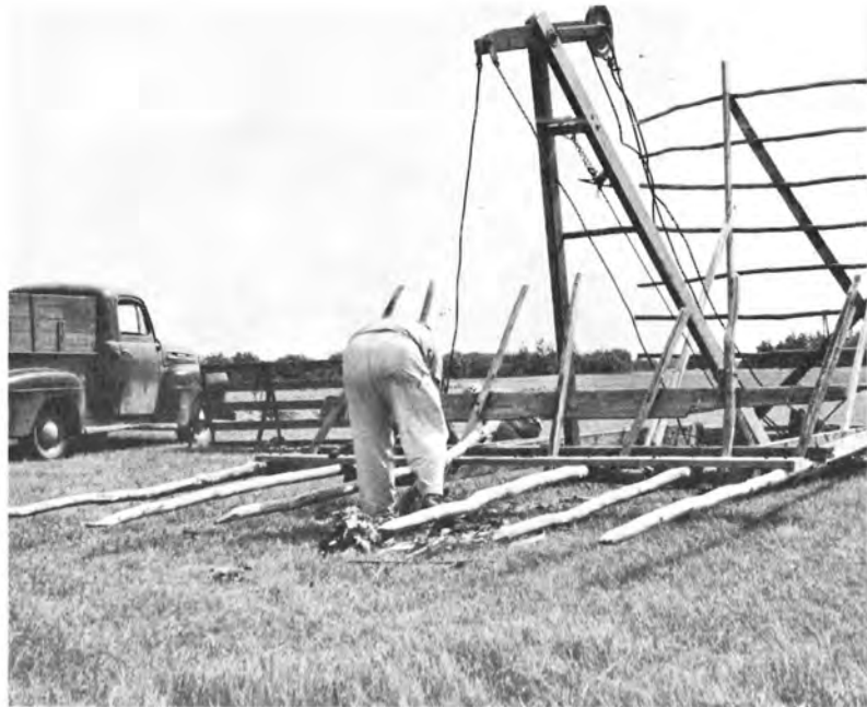
82. Home-made hay stacker by means of which hay was stacked quickly efficiently without the high overhead for expensive machinery
