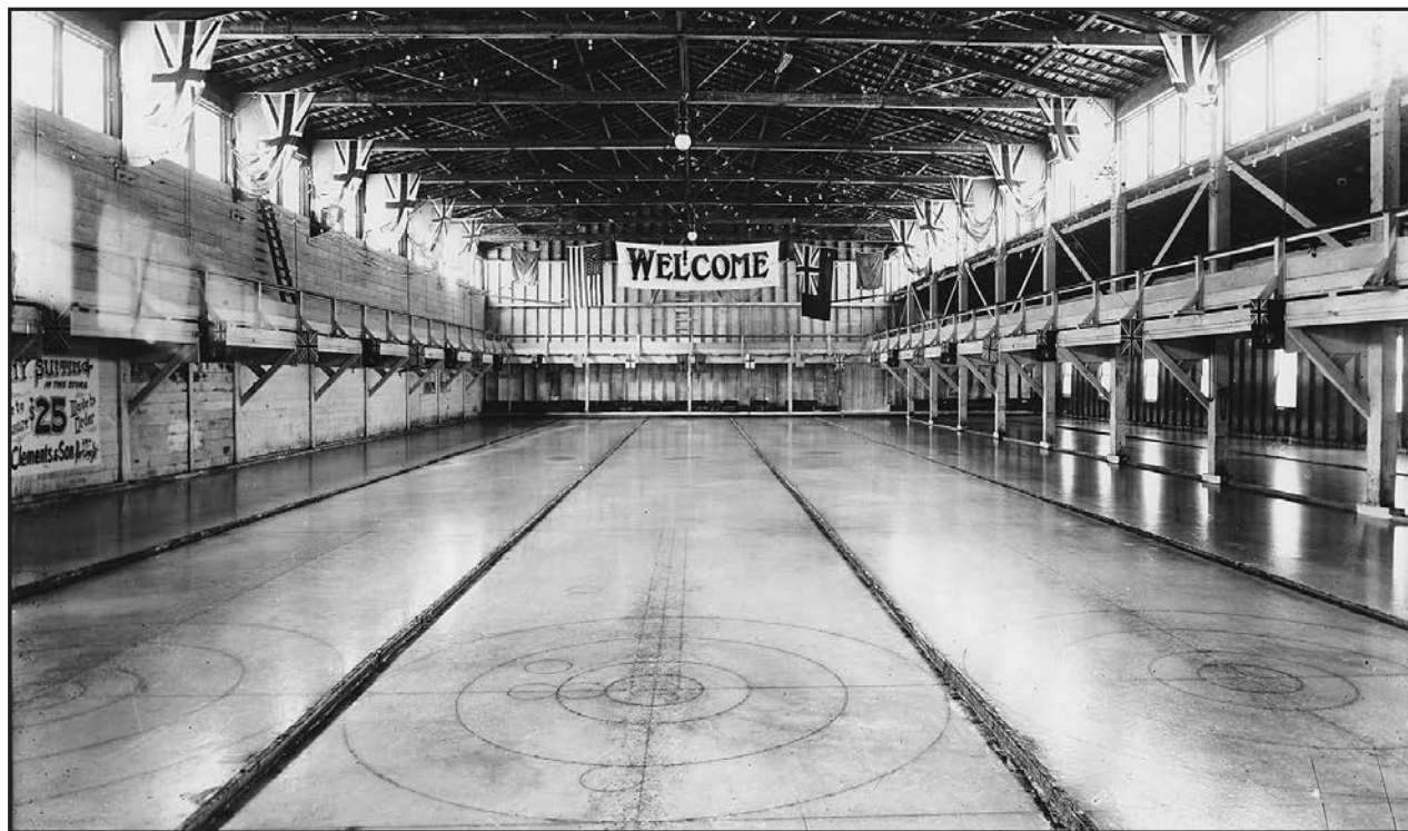
Above: A Lewis B. Foote photograph of Winnipeg's Board of Trade seven-sheet curling rink circa 1915. A wood frame structure with both natural and electrical lighting. Note the two sheets at the right are located in a shed-roof addition with a row of windows at street level. (A. of M. - Foote Coll.)
