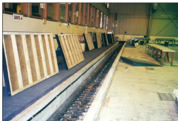
Above: Brine header repairs. 2012.
