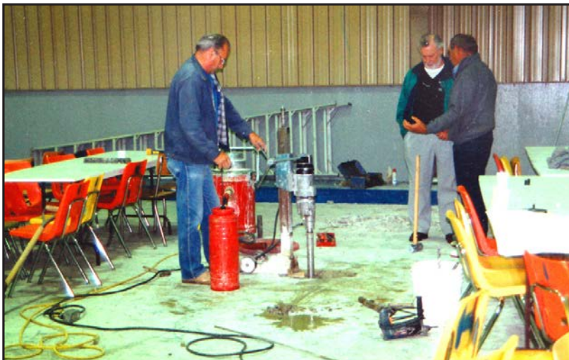
Left: Drilling under sheet 8 in 1992 to test soil moisture levels, which resulted in weeping tile installation to try to address the long-standing problem with uneven ice on that sheet. Len Spitznagel and Walter Perchaylo discussing the matter at right in the photo.
