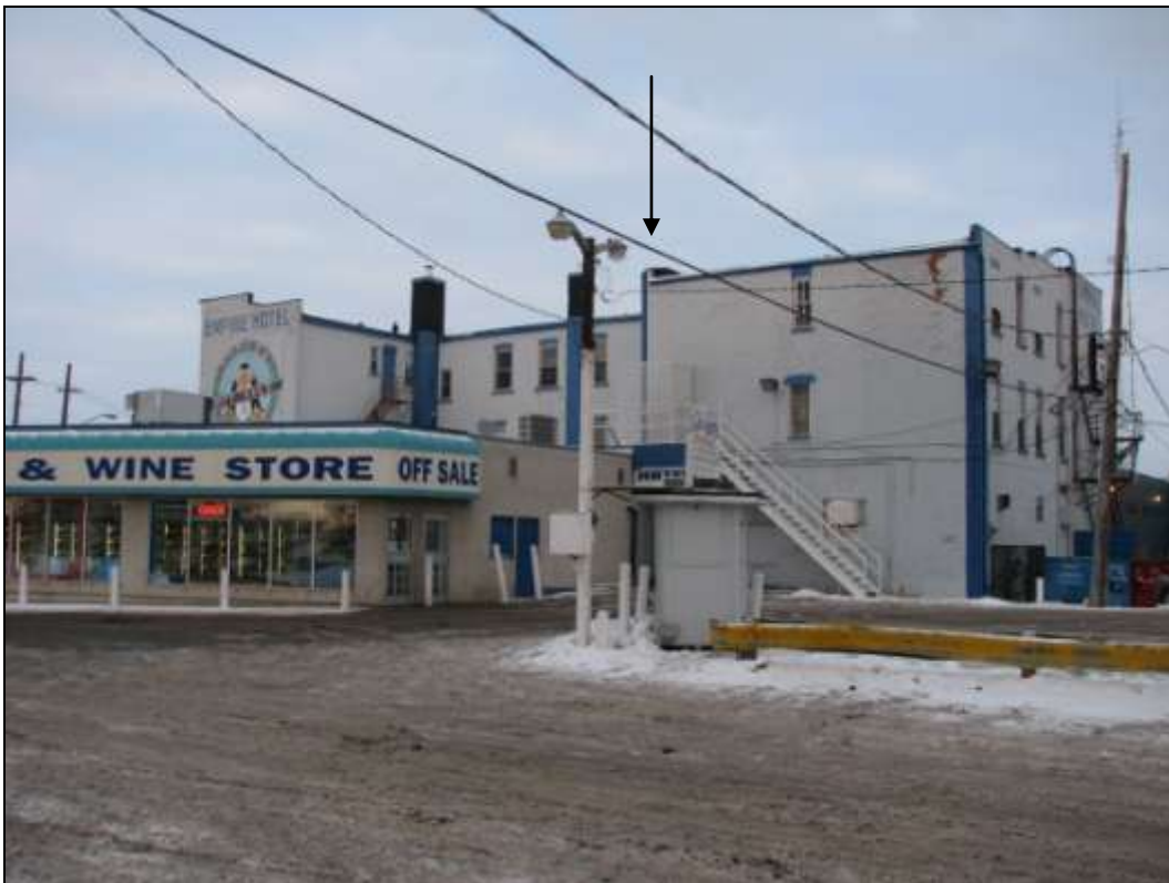
Empire Hotel – West and South sides - 12 January 2008. The south addition is to the right of the arrow. (Source: Frank Korvemaker)
